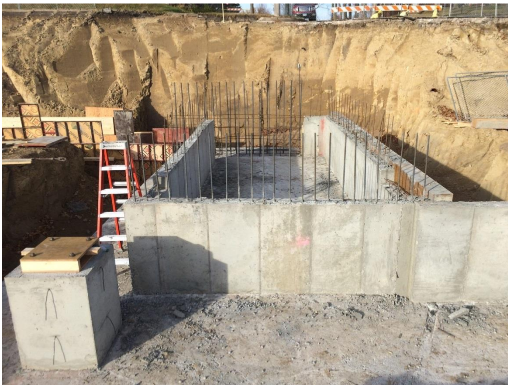
Stair A pad and footing walls poured.
