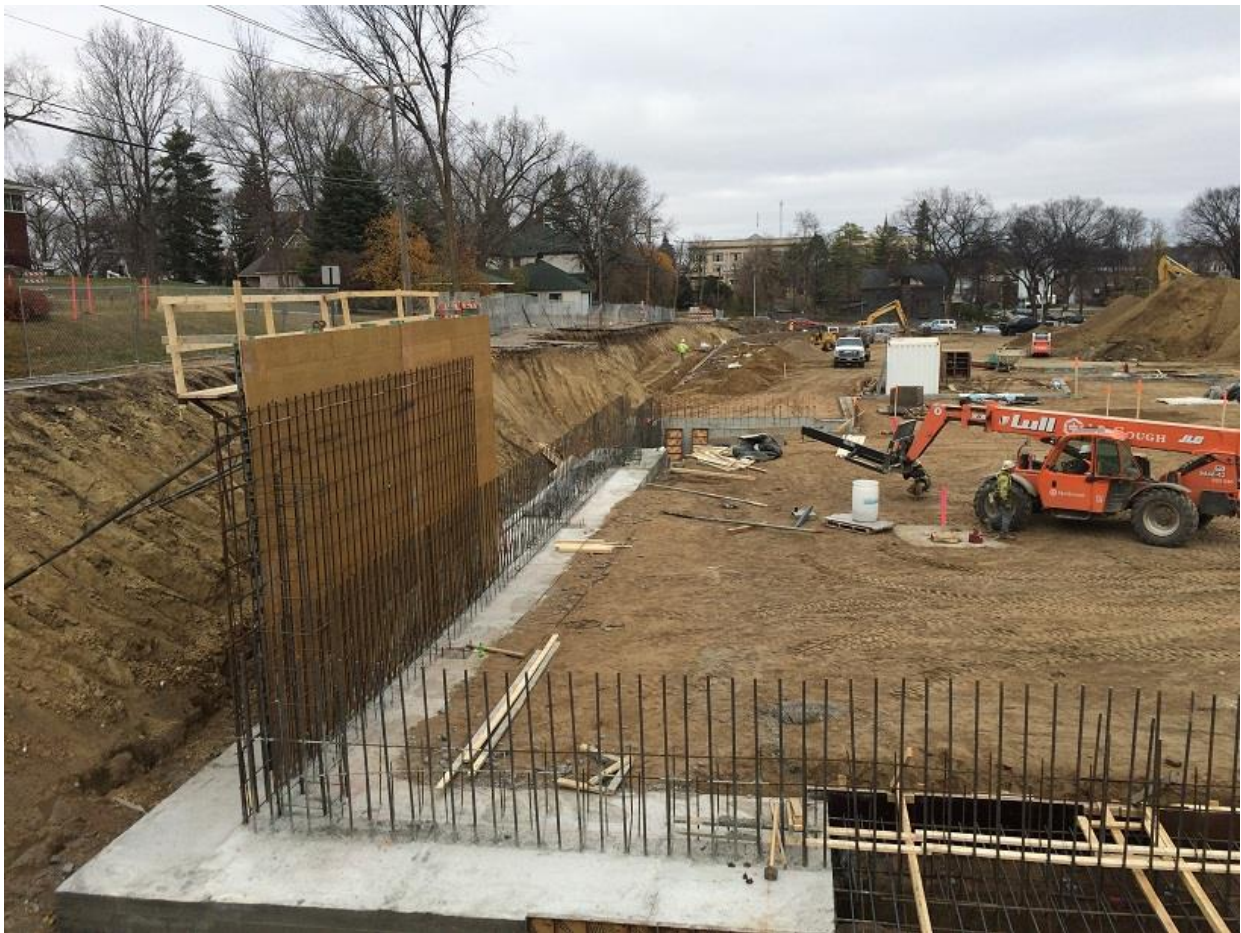
West Footing Poured and Wall forms going up.
