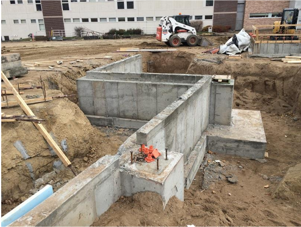
North Footing/foundation walls poured between gridlines 3.7 – 4.6.
