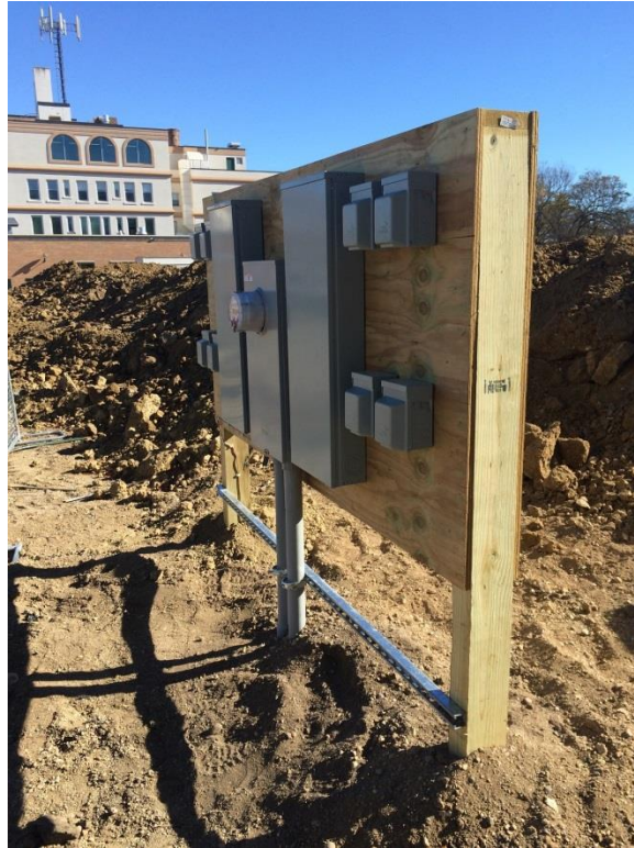
Temp Power Panel Installed and energized.
