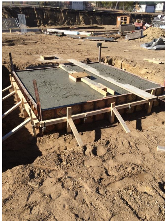
Large Column pad poured.
