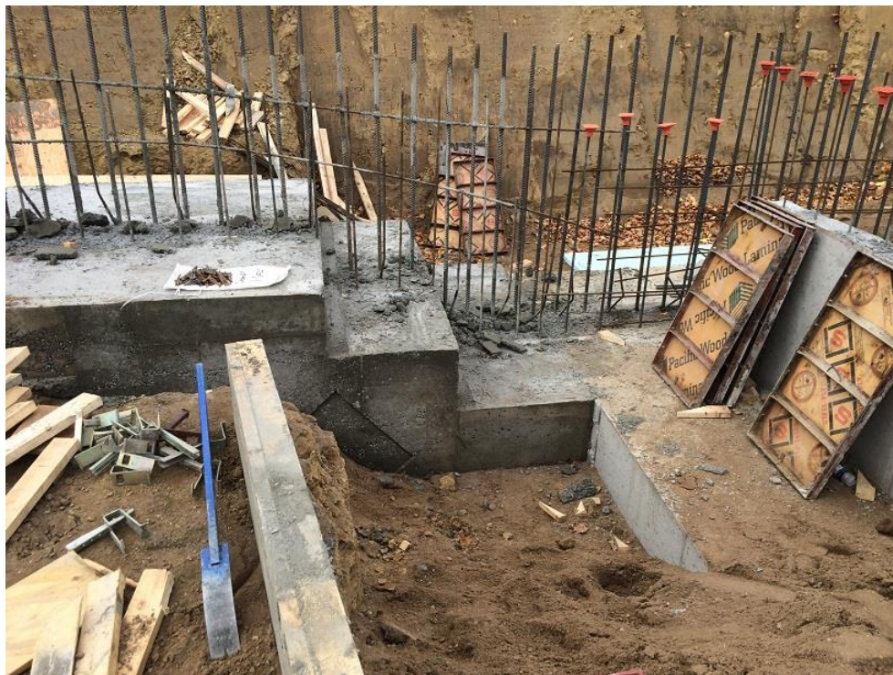
Footing Steps by Stair A.
