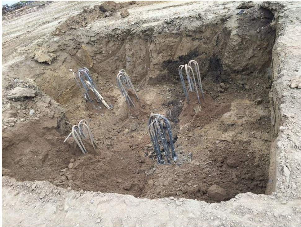
Digging out for Pile Cap.
